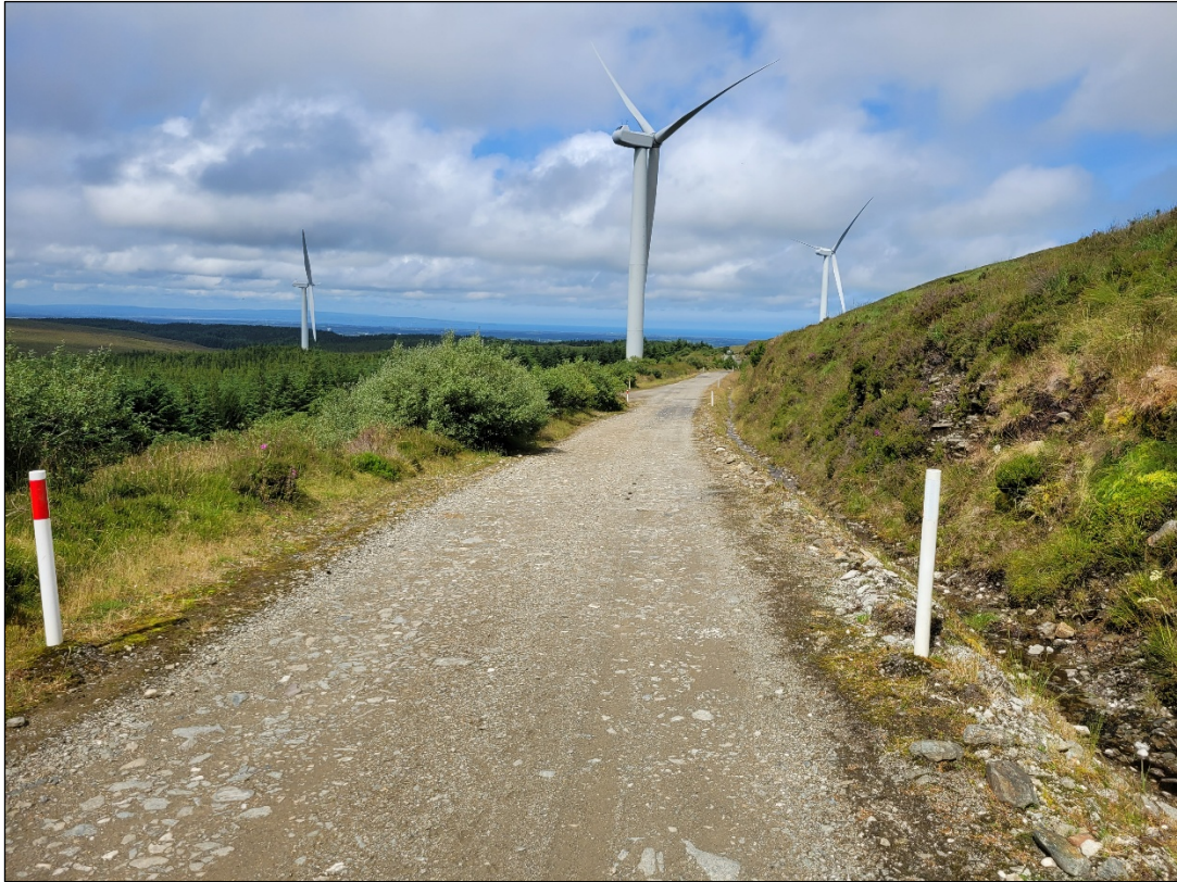
Existing founded access road on east side of site, close to BP3
