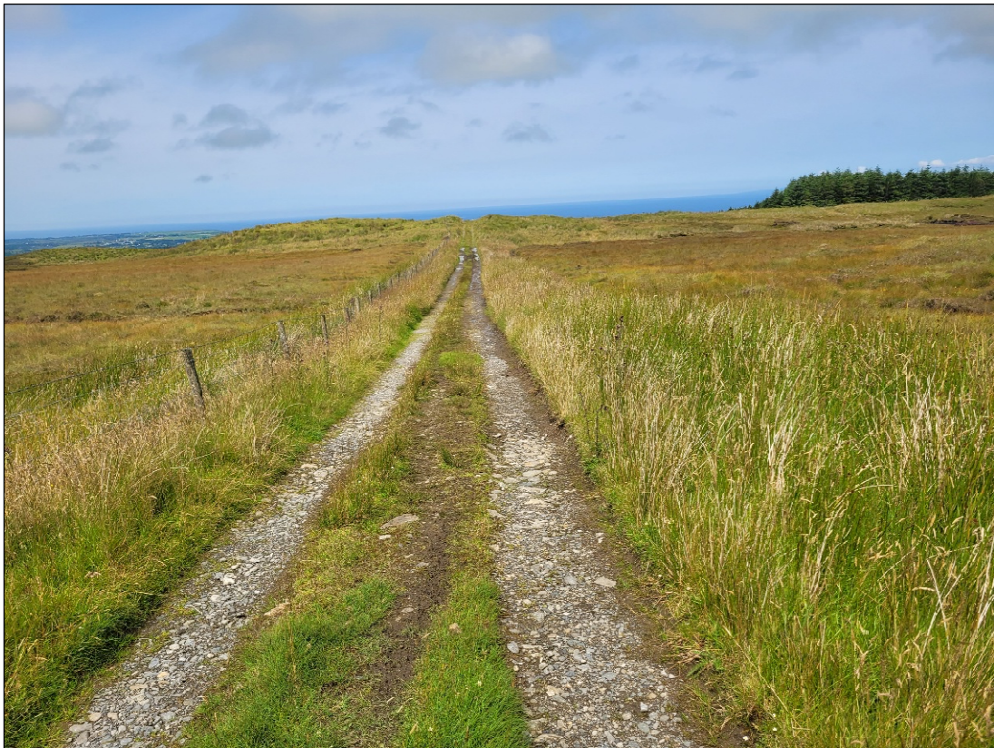
Existing floating access road on site, looking south towards T12
