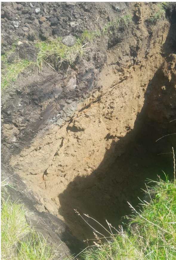
Figure 13 H:\2025\25SO101_EaskyWF\Crumhach (Easky) Windfarm\TP04(2).jpg
