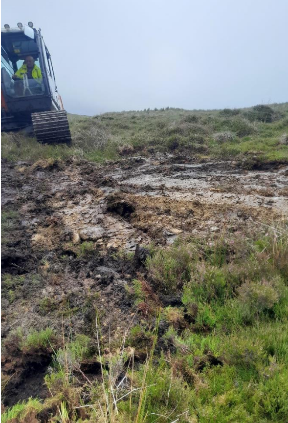
Figure 1 H:\2025\25SO101_EaskyWF\Crumhach (Easky) Windfarm\TP01 (1).jpg
