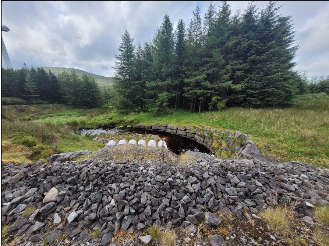
Water crossing on existing wind farm, east of BP3
