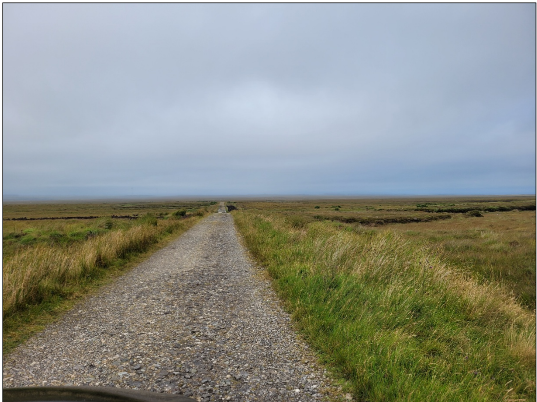
Existing floating road in western section of the Site, close to T05
